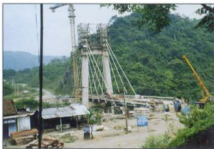
DAKRONG QUANG TRI BRIDGE
